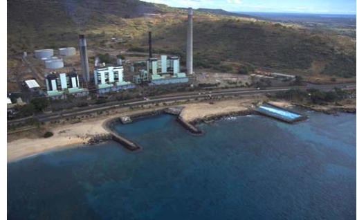
Kahe Power Plant (HECO)
